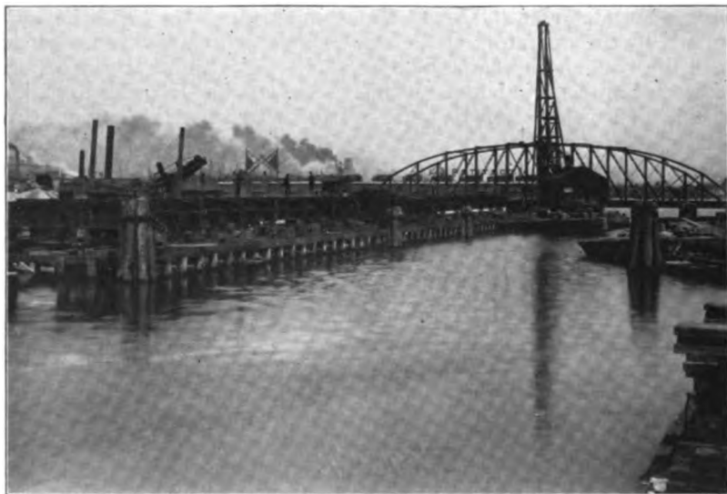
Fig. 17.—Bridge Floor During Erection.
