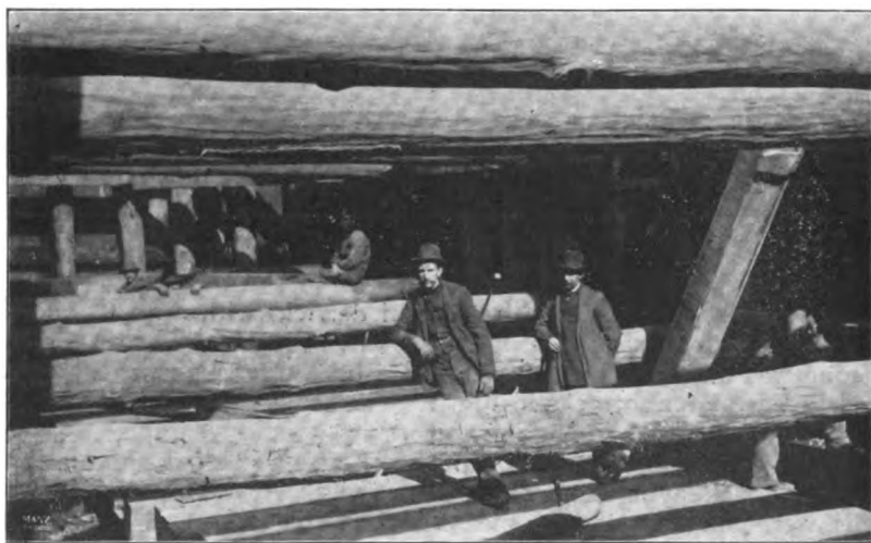
Fig. 8.—Abutment Coffor Dam.
