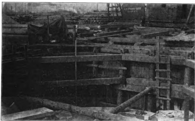
Fig. 7.—Center Pier Coffor Dam.
