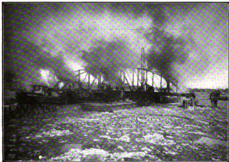
Fig. 5.—The Bridge Being Landed.
